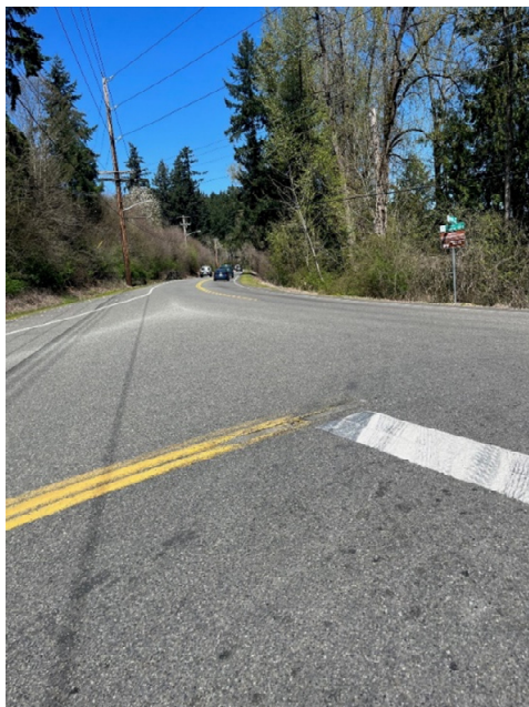
Looking West from Angeline Road
