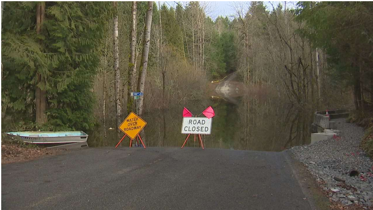
Exhibit 10: Image of 2016 Flooding at 188th Ave E and 62nd St E
