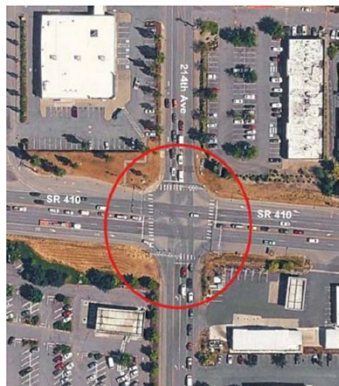
Figure 26. SR 410 at 214th Avenue
