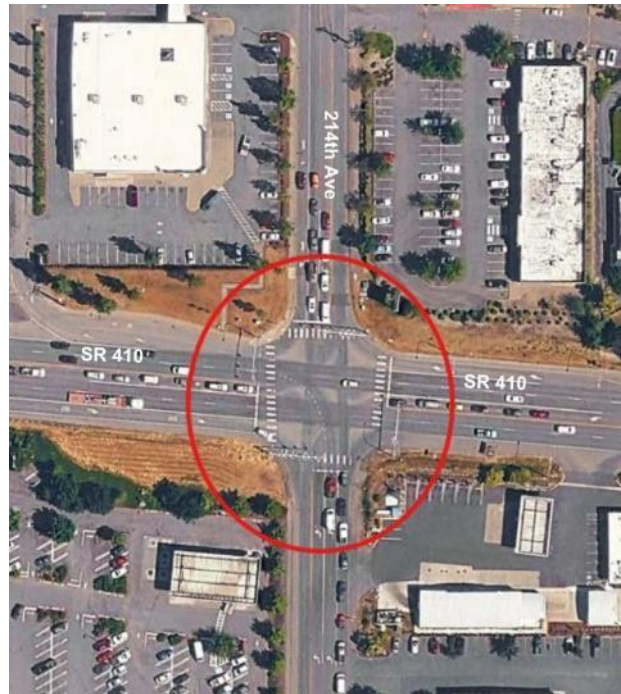
Figure 26. SR 410 at 214th Avenue
