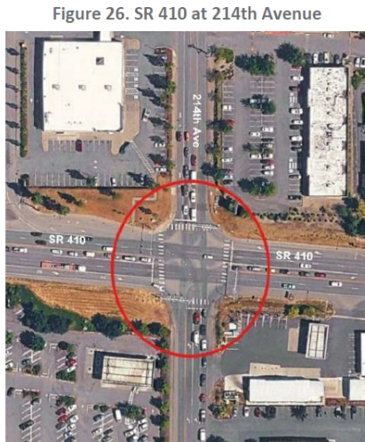
Figure 26. SR 410 at 214th Avenue
