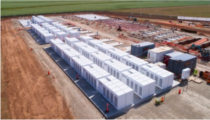
Figure 7: The Hornsdale Power Reserve (South Australia) in the process of expansion from 100 MW/129 MWh to 150 MW/193.5 MWh, as of November 2017.
