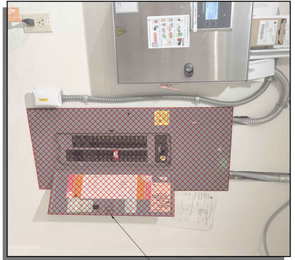
EXISTING LIGHTING PANEL, "E-LP" TO BE REMOVED
