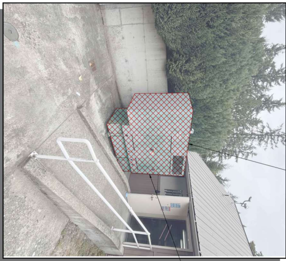
CUT AND CAP EXISTING CONDUITS AT GRADE.
