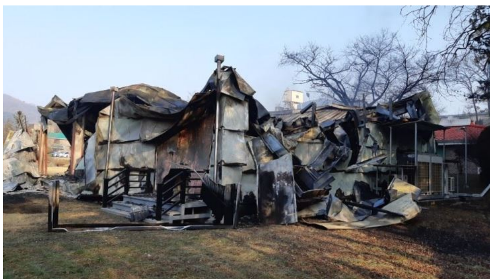
Figure 2: Remains of a Korean BESS destroyed by a “battery fire”. An energy storage system was destroyed at the Asia Cement plant in Jecheon, North Chungcheong Province, on Dec. 17. Courtesy of North Chungcheong Province Fire Service Headquarters (Korea Times 2 May 2019)
